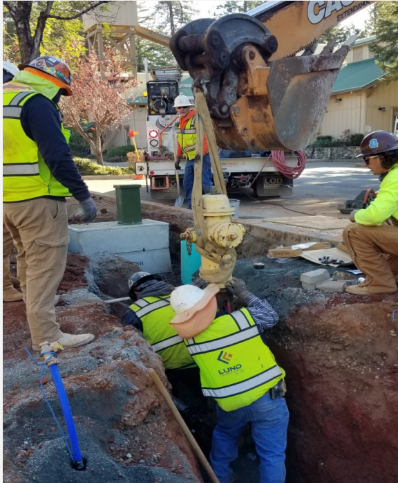
Installing Fire Hydrant
